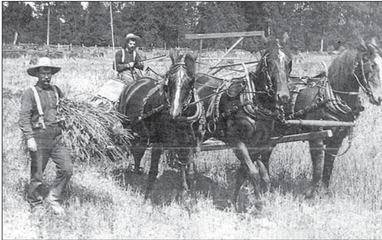
The earliest reapers cut stalks of grain, depositing them at the side of the machine.
