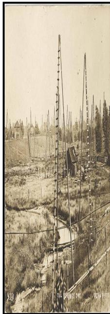
With the introduction of steam engines, the weight of drill bits could be considerably heavier than for spring pole systems. Cable tools were particularly suitable for drilling medium hard rocks. By the turn of the century cable tools, under favourable conditions, could complete wells down to about 900 m. The first drilled oil well in Canada was completed in 1859 by James Williams using a spring pole at Oil Springs to tap an oil reservoir at a depth of 50 m.
