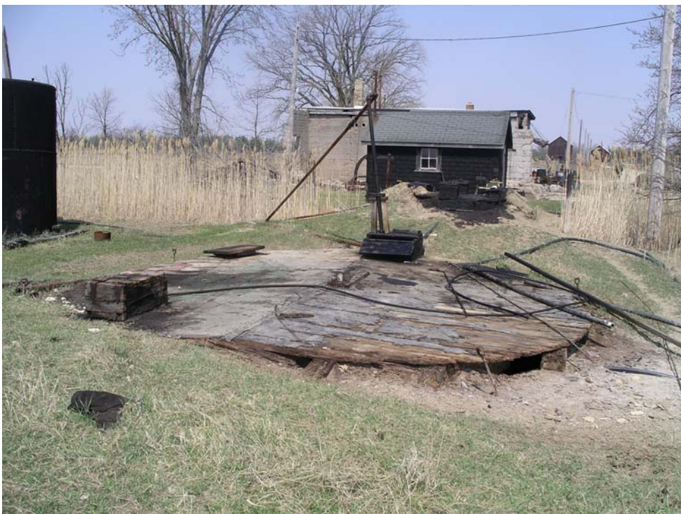
Figure 15. Below-grade wooden oil tank – Oil Springs. ( A. Roos, Parks Canada, April 2005 )
