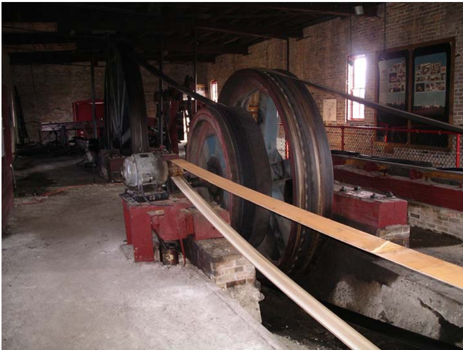
Figure 13. Machinery inside rig house – Oil Springs. ( A. Roos, Parks Canada, April 2005 )
