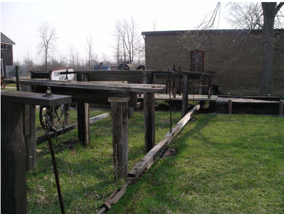
Figure 19. Operational rig building with jerker lines coming out of the building – Petrolia Oil Museum. ( A. Roos, Parks Canada, April 2005 )
