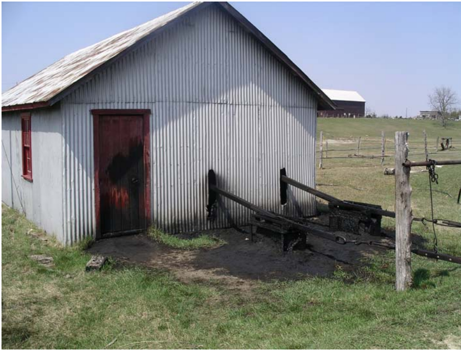
Figure 12. Rig house with jerker lines coming out from machinery located inside – Oil Springs. ( A. Roos, Parks Canada, April 2005 )
