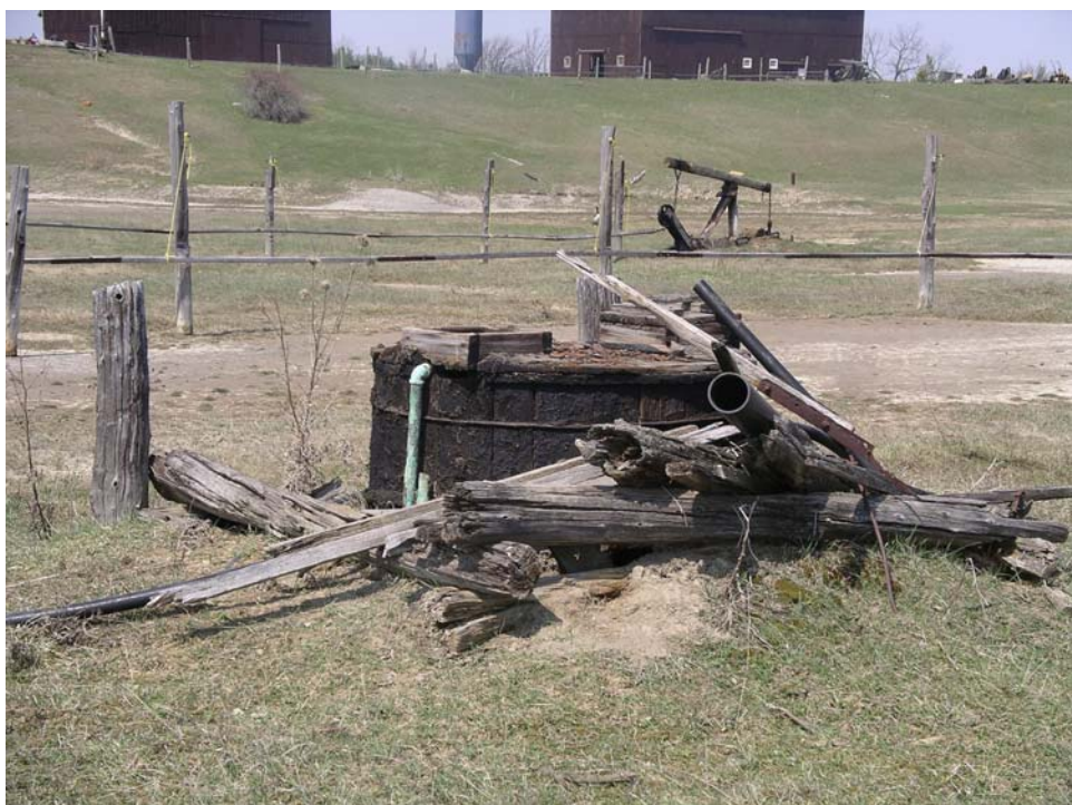
Figure 8. Williams-dug oil well near the museum with a three-pole derrick – Oil Springs. (A. Roos, Parks Canada, April 2005)
